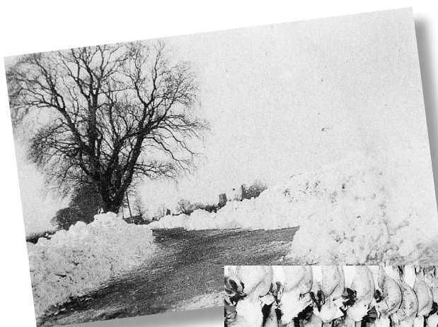
1 Church End looking back into the village c 1954
